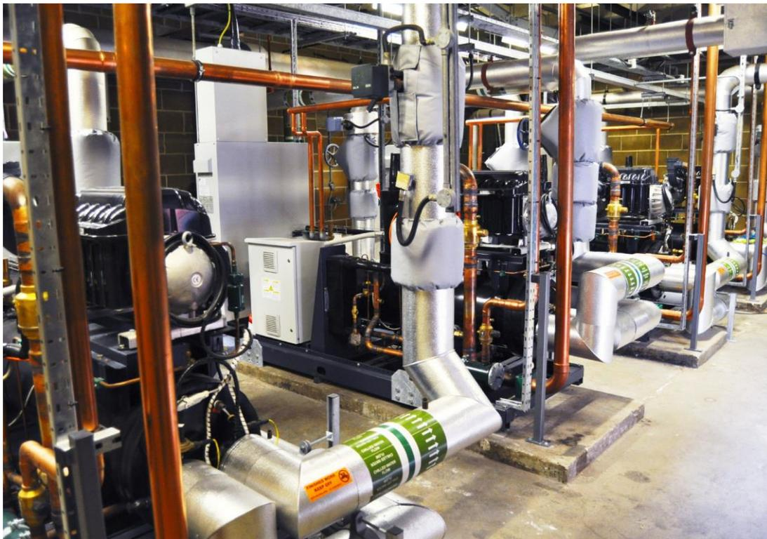
The high efficiency R134a-based chillers replace four aging R22-based Hitachi units, on dual screw compressors, believed to be up to 20 years old. The Turbomisers were installed on the existing mounting points, however they occupy two-thirds the space, due to their high performance relative to their size.
