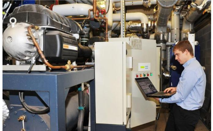
Connection requires the end user's permission, but once authorisation is given enables engineers to monitor plant performance remotely, and diagnose potential problems prior to – or overcoming the need for - a site visit.
