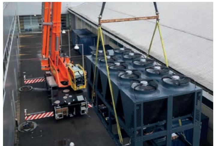
The project was a full turn-key package which included removing the existing chiller and single fixed speed pump and replacing with a new chiller and inverter pump set for redundancy should a pump require maintenance. All this had to be carried out in the shortest possible time frame to reduce the chilled water downtime as to not affect the Olympic athletes. To minimise the shutdown Cooltherm suggested the work was carried out over 2 short shutdown periods rather than one extended one.
