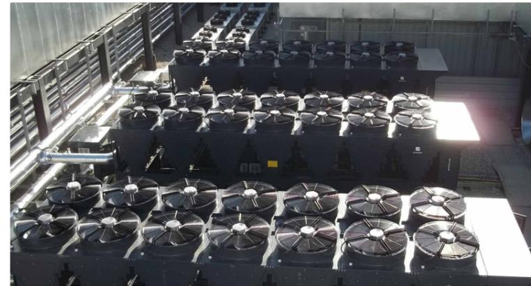
each chiller Cooltherm devised an alignment bracketry arrangement that allowed the second section of chiller to swiftly align with the first with ease, then a series of pin guides ensured the chilled water pipework and cable containment met within a tolerance of 2mm of each other between chiller sections.
