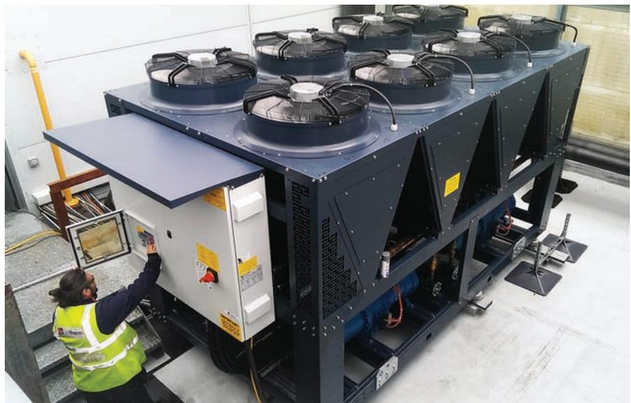
**Figure 1: A 500kW air-cooled propane chiller (Source: Cool-Therm)**
